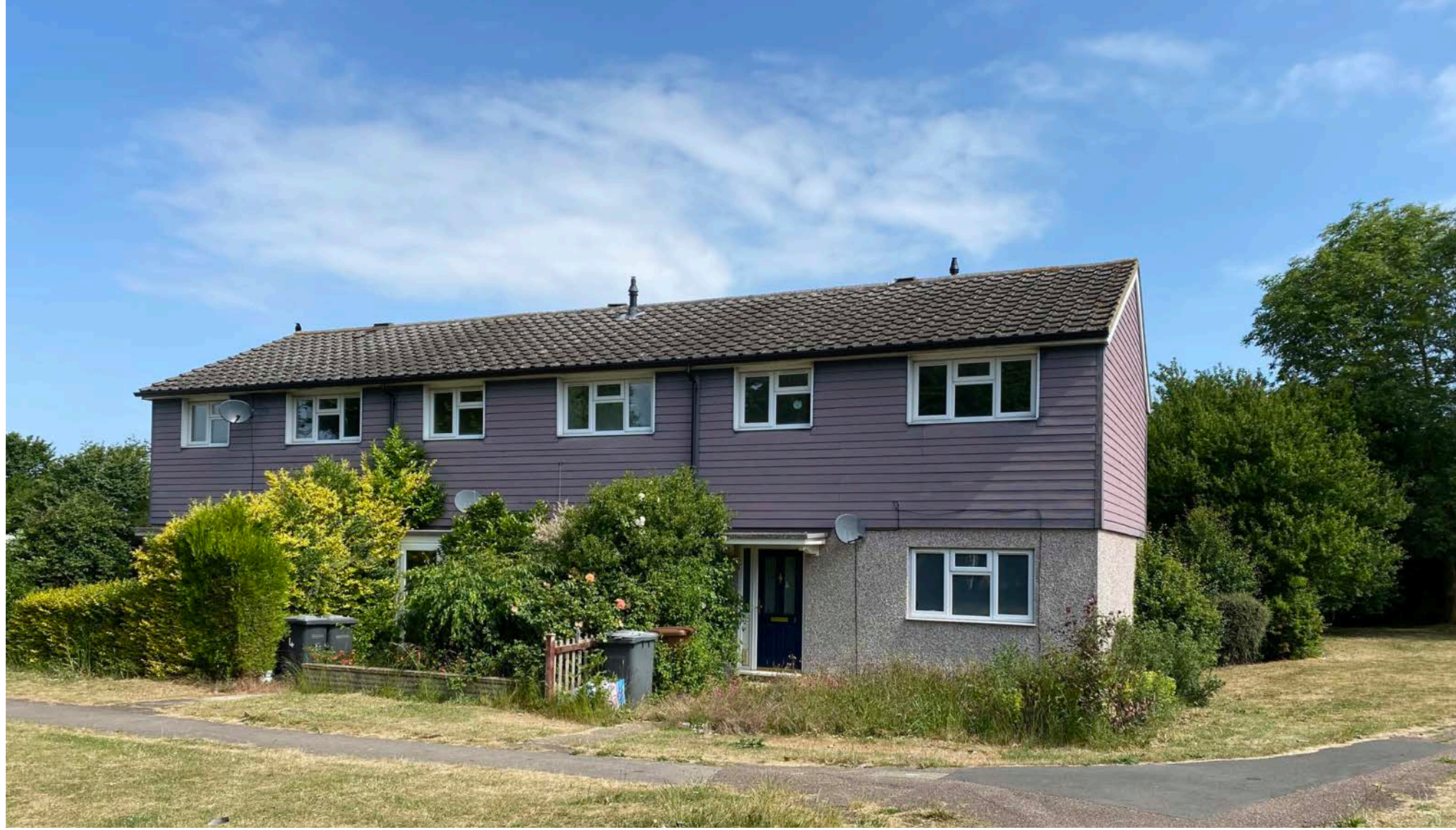
Existing site photograph
