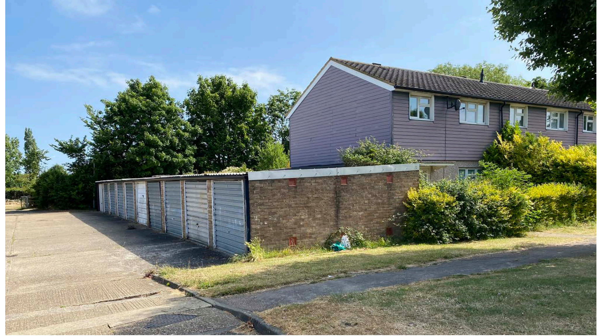
Existing site photograph showing garages and access to rear allotment site
