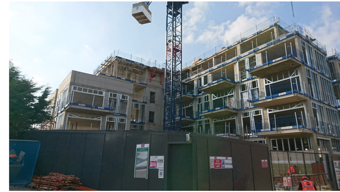
Photo of current site progress at Phase 1
