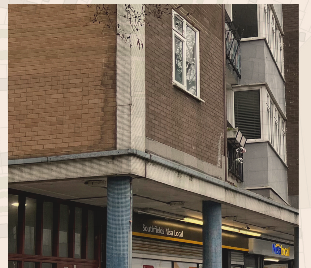
Limited insulation provision resulting in low building quality.
