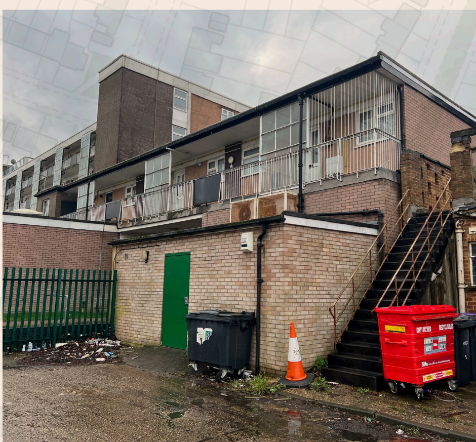
Service zones dominating street elevations creating poor/undesirable views across the area.
