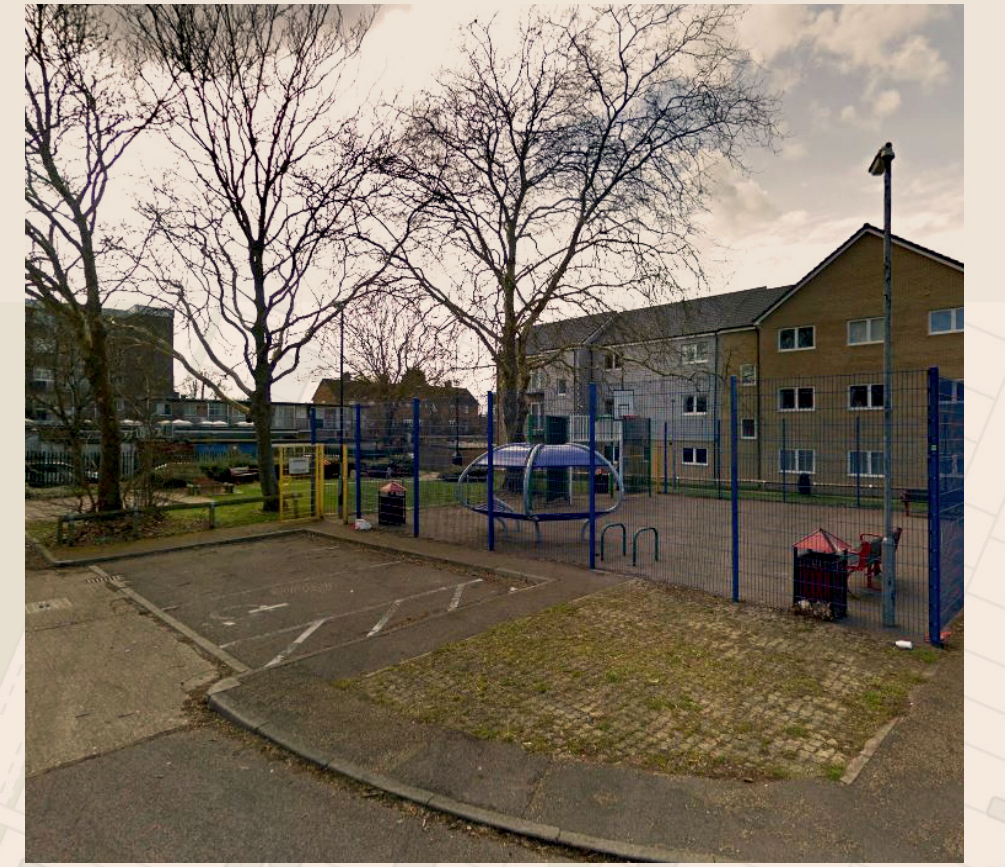
Pavements being 'cut-off' by street parking bays and damaged grass verge.
