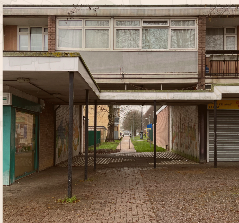
Pedestrian route cutting through service areas, creating dark and unattractive spaces - lack of sense of community.
