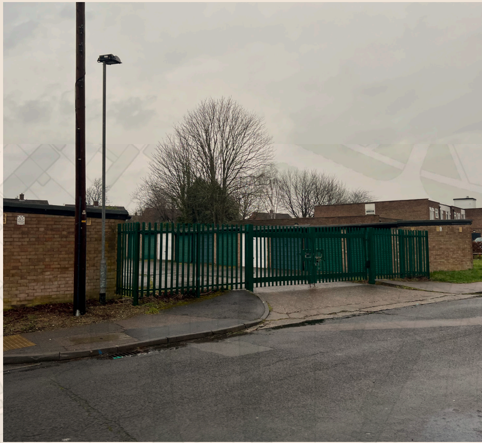
Buildings with no windows and fencing to street frontages leading to security issues, lacking natural surveillance.
