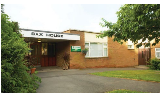
SAX HOUSE Western Close, Letchworth, SG6 4TA
